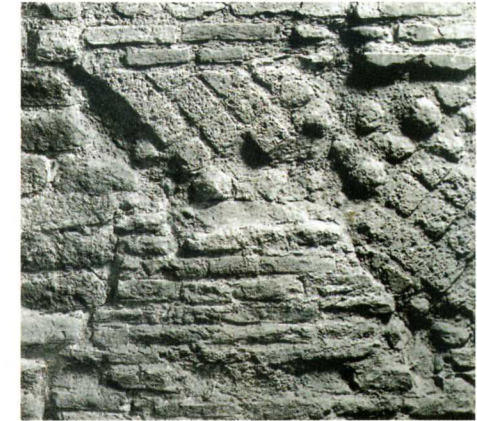
Muro in opus mixtum
